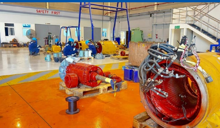
Various alternator servicing and rewinding work in our newly fitted out workshop
